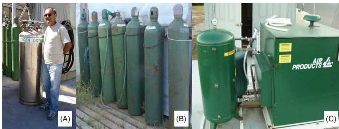
FIG. 5.11 Pure oxygen supply; (A) Liquid oxygen bottle (LOX), (B) Compressed oxygen cylinders, (C) Oxygen generator.
