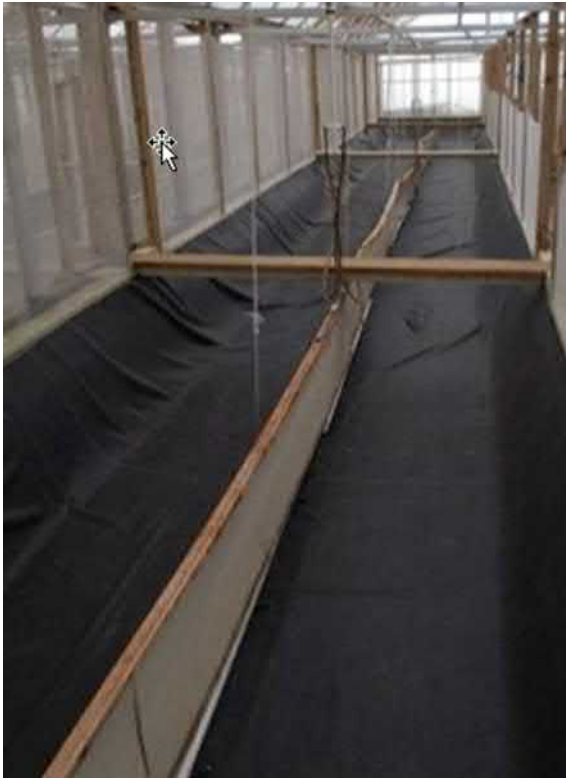
FIG. 5.3C Raceway lined with EPDM membrane.
