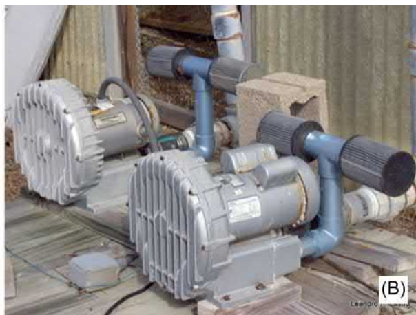
FIG. 5.6 Positive displacement blower with belt drive (A) and regenerative blowers (B) driving diffusers and airlifts in the Texas A&M-ARML 40 m 3 raceways. Blowers have inlet filters.
