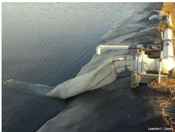
FIG. 6.1 Filter bag on seawater inlet of Texas A&M-AgriLife Research Mariculture Lab.
