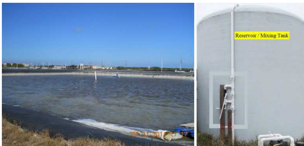
FIG. 5.1 A 2500-m 3 reservoir pond (left) and 36-m 3 mixing tank (right) at the Texas A&M-ARML.
