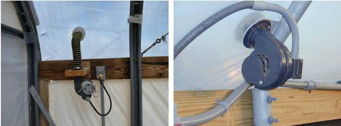
FIG. 5.3 Air blowers inflate double-layer polyethylene greenhouse roofs at the Texas A&M-ARML.
