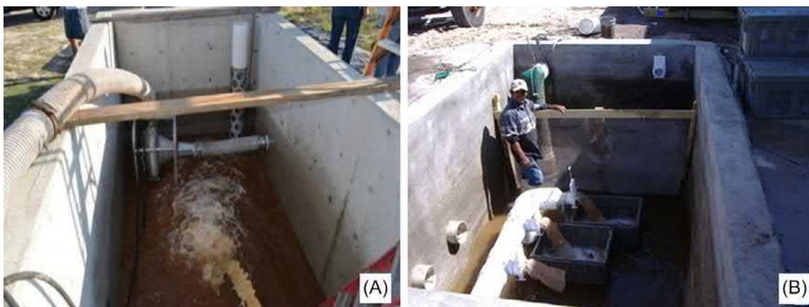
FIG. 5.2 Concrete harvest basins at the Texas A&M-ARML (A) and at Bowers Shrimp Farm, Palacios, Texas, US (B). (Photo by Tim Morris, Bowers Shrimp. Used with permission.)
