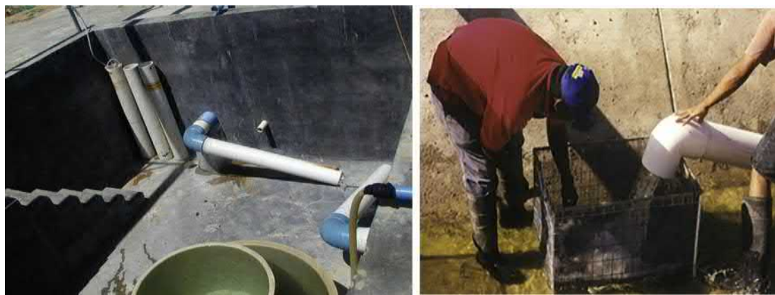
FIG. 8.20 Harvest by swivel standpipe.
