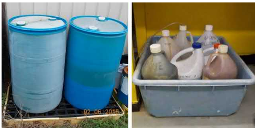
FIG. 6.5 Chemical storage in containment trays to limit spills.
