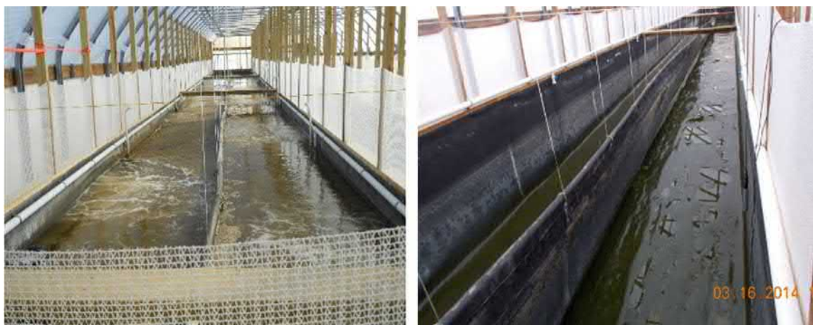
FIG.5.43 A full and empty raceway. Notice freeboard in the full raceway.
