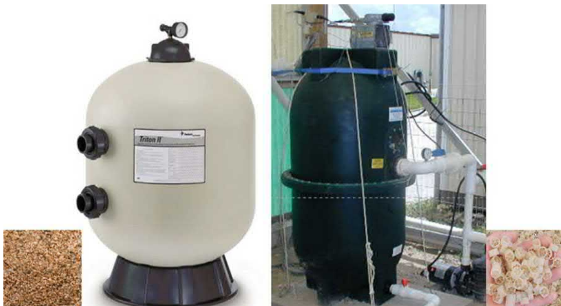
FIG. 5.16 Left photo—Pressurized Sand Filter with sand used for filtration; Right photo—Poly Geyser bead filter with bead media.
