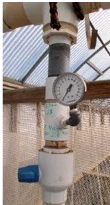
FIG. 5.5 Air pressure gauge. Note installation of a 5-cm PVC valve for pressure regulation.
