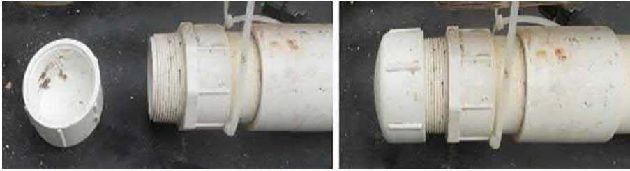
FIG. 9.2 The 5-cm PVC screw cap of the bottom spray pipe at the raceway's deep end.
