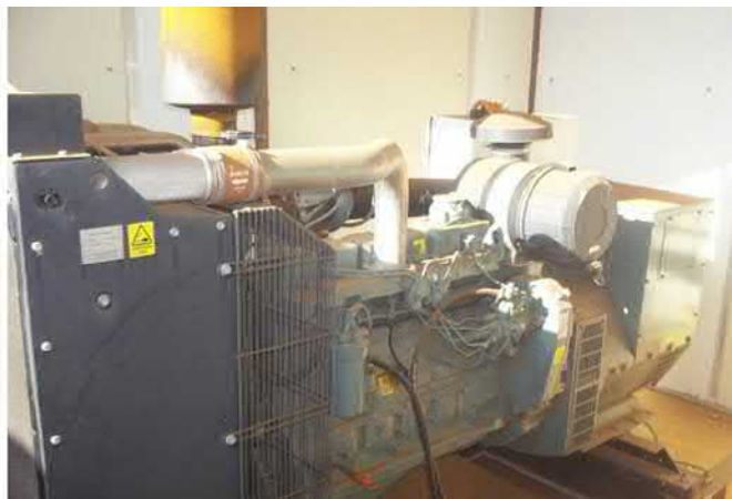
FIG. 5.4 Backup diesel generators (30kW and 250kW) installed at aquaculture facilities.
