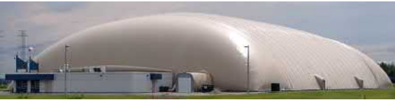
FIG. 5.1C Inflated air-supported structure (Photo by Wikipedia. Used with permission)
